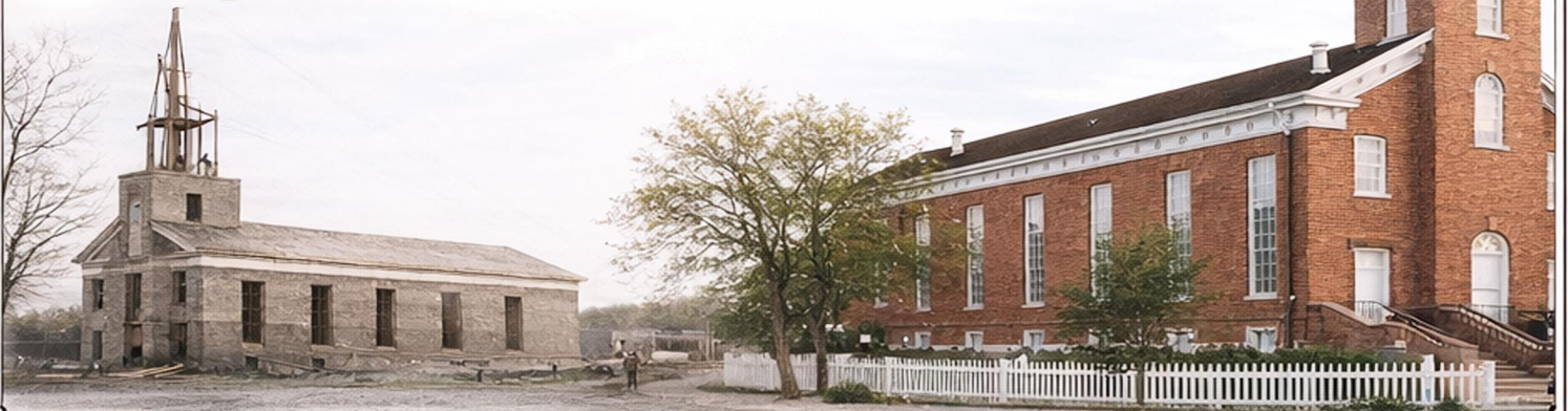
St. George Tabernacle during construction, late 19th century.
